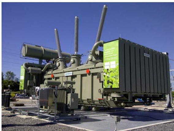
Fig. 4 Siemens 420 kV extra-high voltage power transformer filled with Natural ester liquid
